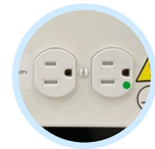
Hospital grade electrical receptacle
