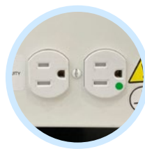
Hospital grade electrical receptacle
