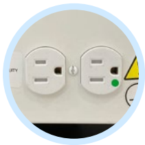
Hospital grade electrical receptacle
